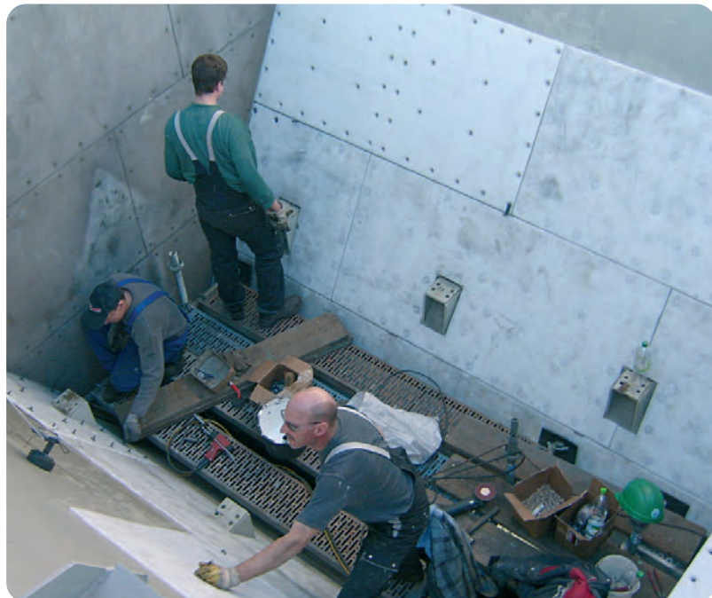
Stud-welding process: lining a hopper
